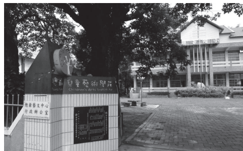
Figure 5 The Previous Condition of the Tsung-Yeh Elementary School Source: the author Date: September 6, 2013
